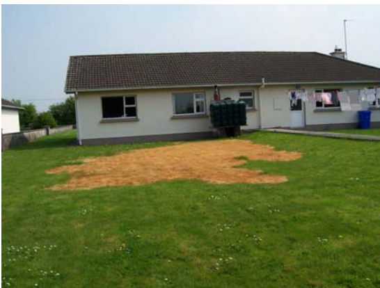
Heating oil spill has damaged the lawn
