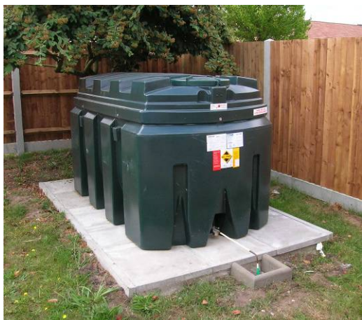
Correctly installed domestic oil tank
